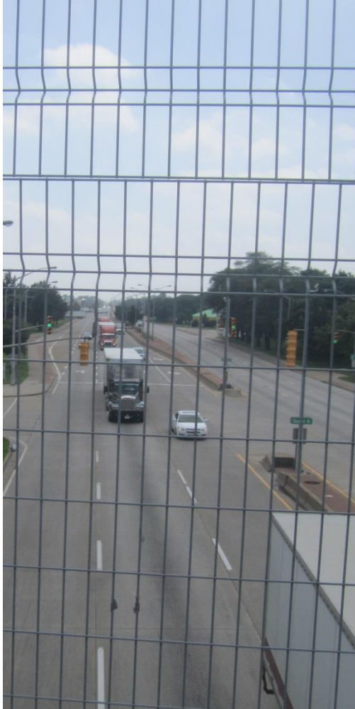
Huron Church Rd. Approaching the Ambassador Bridge, Windsor
